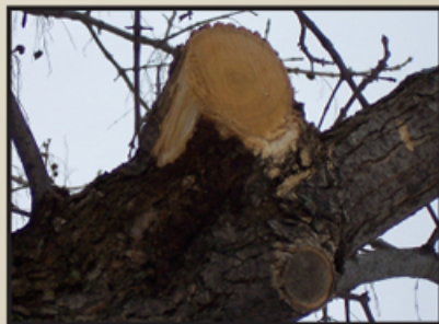
Stub Cut & Tear Cut
