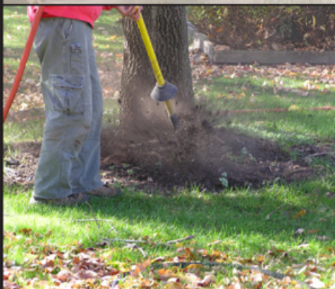
Top soil is blown away using an Air Spade™ tool
